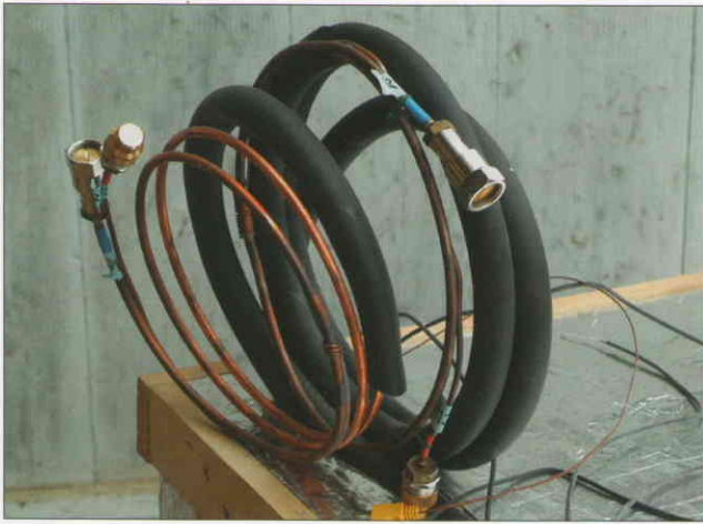
Left —Precharged refrigerant lines. The installer has only to screw the various system components together ( right ); no vacuuming-down or charging with refrigerant is required.
