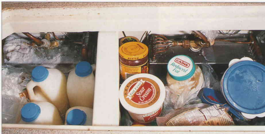
Loaded iceboxes with holding plates (freezer on the left, refrigerator on the right) on the author's previous boat. These boxes have holding plates located at the backs of the boxes. Note the considerable volume they occupy.
